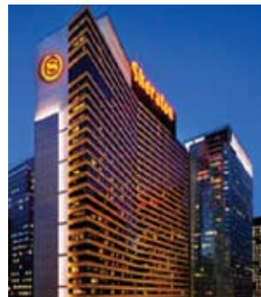
Sheraton New York Hotel and Towers
